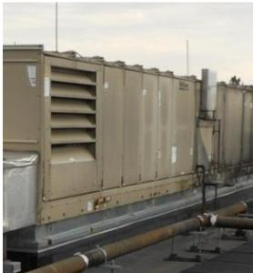
Figure 5: One of nine Rooftop Air Handling Units
